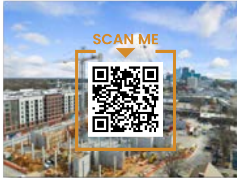
CONSTRUCTION DRONE VIDEO
